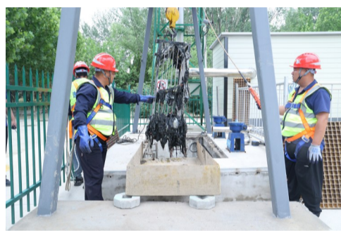
污水泵站应急处置
